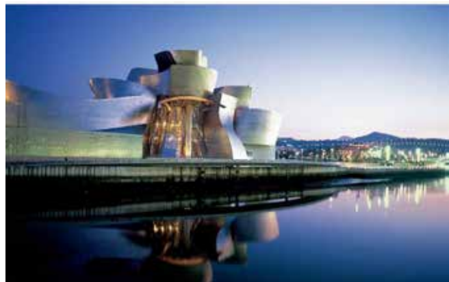
Fig. 4. Guggenheim Museum Bilbao (1997). Canada. Architect. Frank Gery
